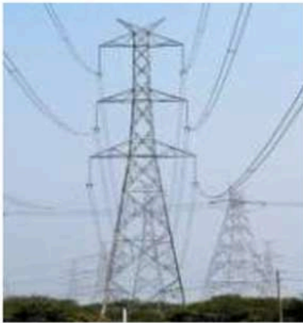
State power utilities owed power generators $6.78 billion.
