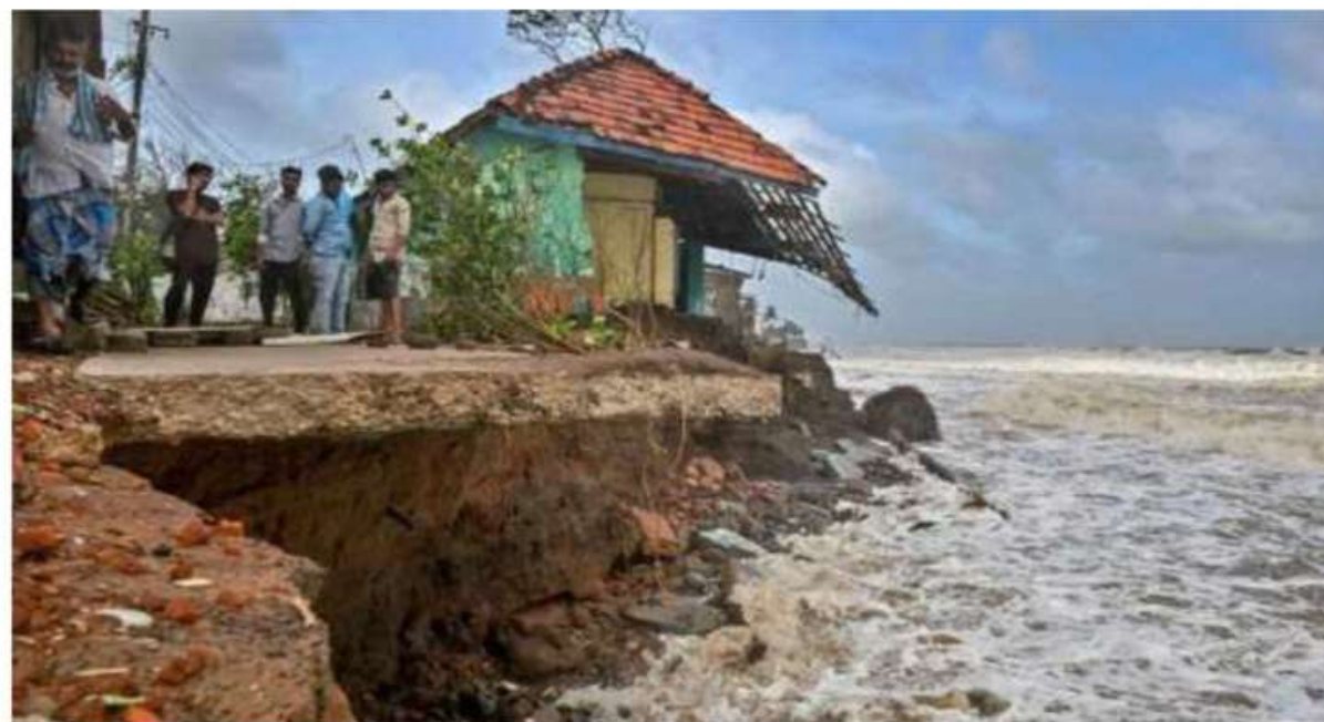
A house damaged by high tidal waves in Kakinada district of Andhra Pradesh on Tuesday. K.R. DEEPAK
