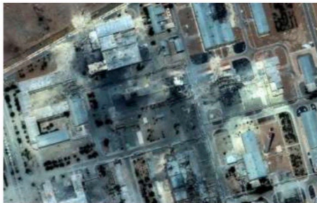
Destroyed buildings at Isfahan Nuclear Technology Centre after it was hit by U.S. air strikes, in Isfahan, Iran, on June 22, 2025. REUTERS
