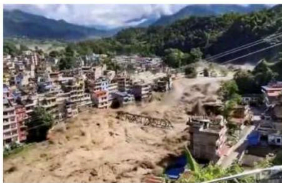
Flood fury: A screenshot shows water flowing across a residential area and damaging a bridge near the Nepal-Tibet border. PTI
